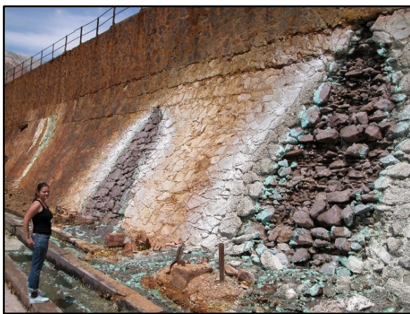
1.a. Retaining dike.
