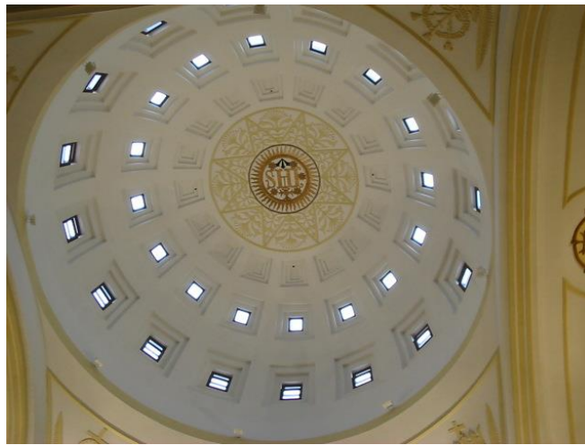
Figure 8. Interior of the illuminated dome of St. Joseph in Macau. Source: Cabeza-Lainez.
