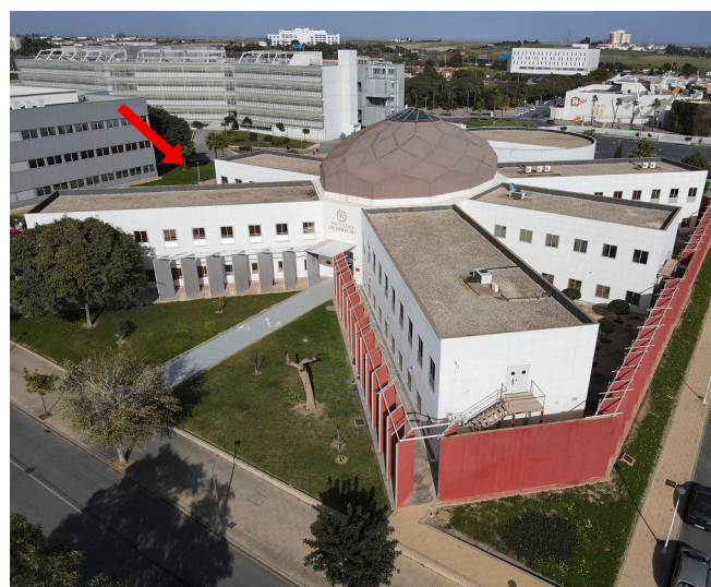
Fig. 1. Building surveyed, located in the city of Huelva (Spain) (The area studied on the building is marked with a red arrow).
