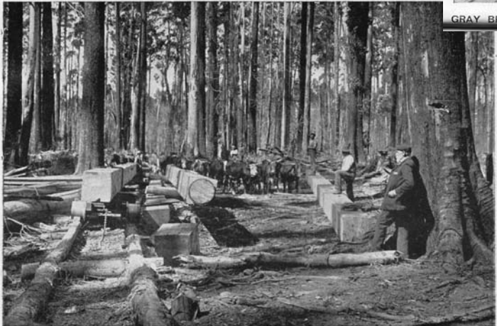
GRAY BROS. PILES READY FOR TRANSPORT ON TRAM, TAFANNA, TASMANIA.
