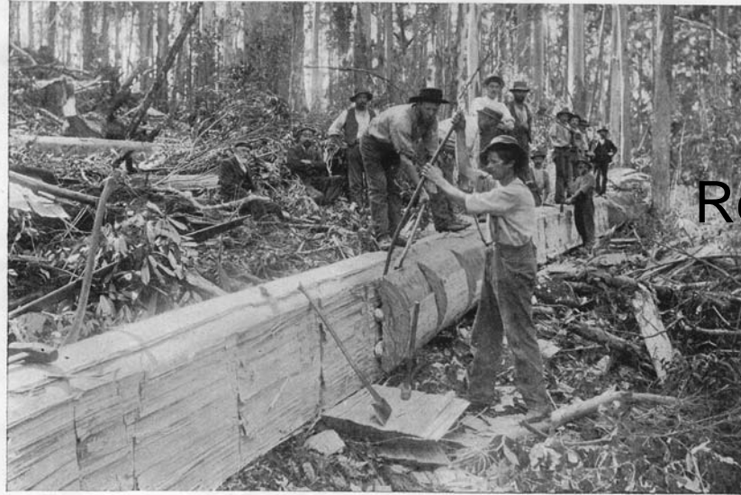
GRAY BROS. SQUARING PILES FOR DOVER (ENG.) HARBOUR WORKS, TASMAN PENINSULA, TASMANIA.
