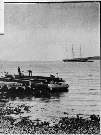
GRAY BROS. Loading Piles for Shipment to South Africa, at Flinders Bay, Southern Tasmania.
