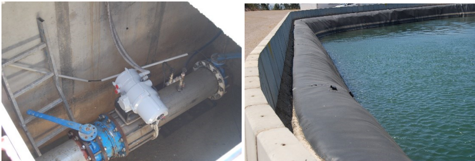
124 Figure 2. Multistream DN300 electrical regulatory valve (Multinar), which controls the flow at the 125 inlet of the WWTP in 'Puebla de Guzmán' (Huelva, Spain) (on the left) and 'Cabeza del Pasto' 126 reservoir which channels water to the WWTP in 'Puebla de Guzmán' (Huelva, Spain) (on the right) 127
