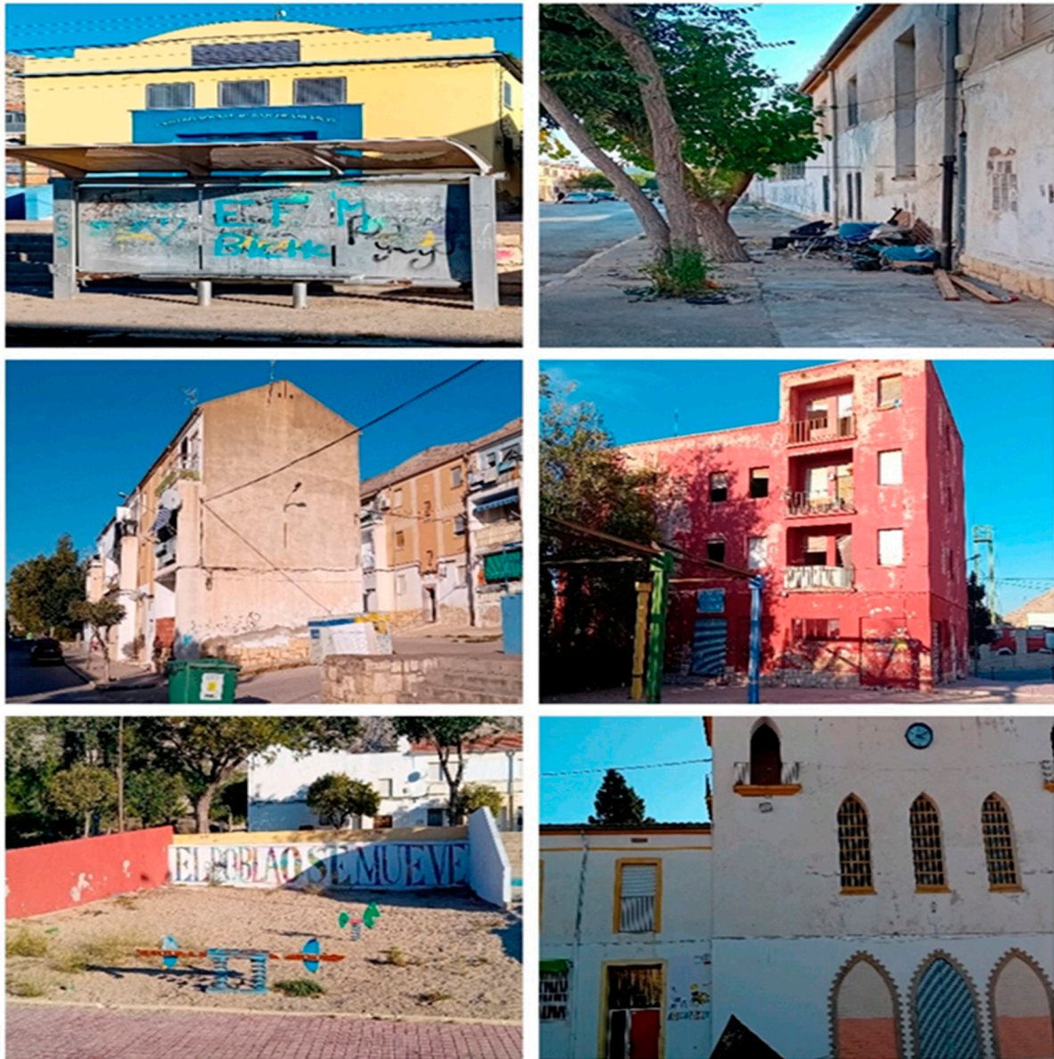
Figure 8. State of deterioration of the neighbourhood housing and public facilities. Source: [44].
