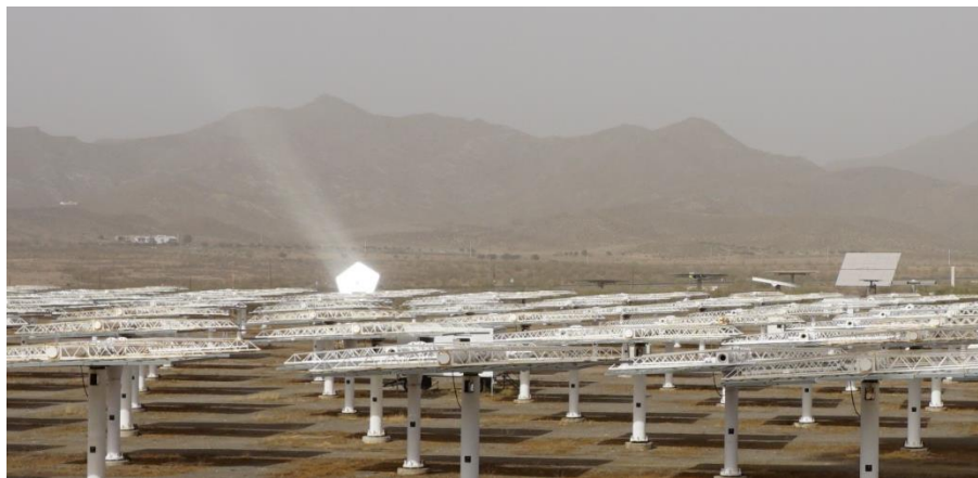
81 Fig. 1: Low visibility and substantial light scattered by large particles in the atmosphere at 82 PSA on 2016-02-22 at 14:30 local time. Solar radiation reflected by the heliostats is visibly 83 attenuated by scattering. 84
