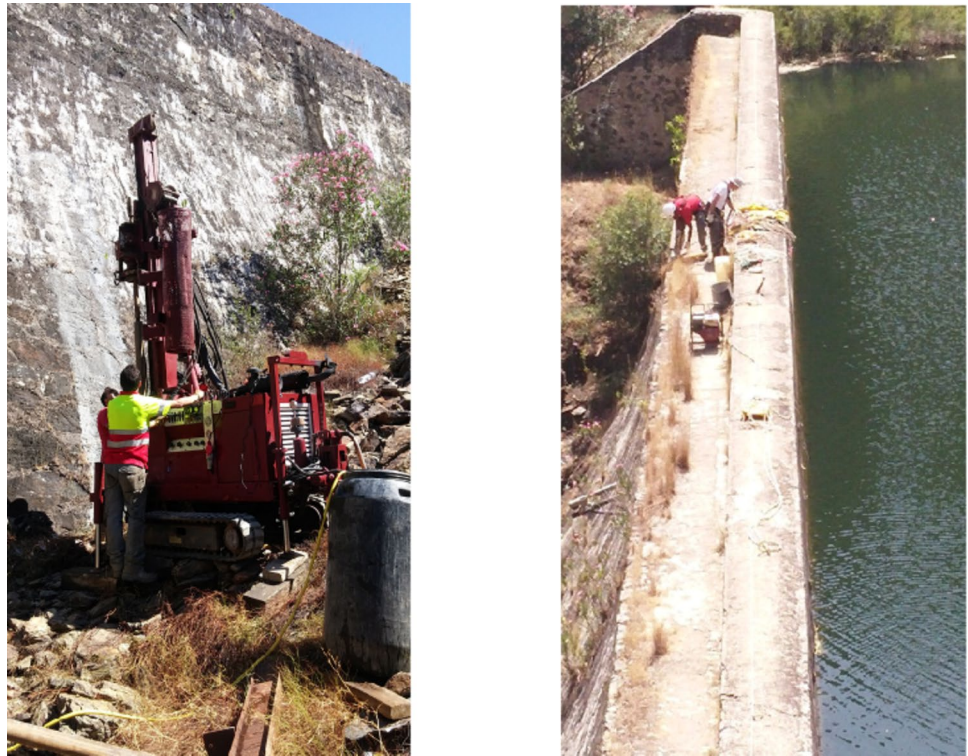
Fig. 12 Detail of drilling machine and core collection at the Calabazar Dam
