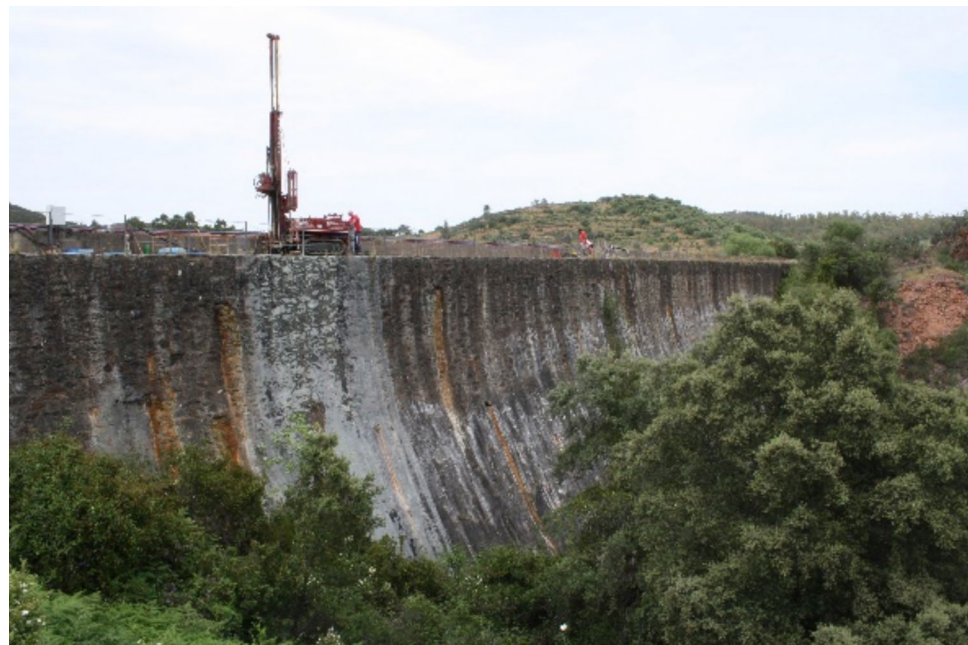
Fig. 4 View of the Alisal Dam
