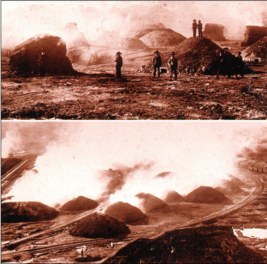
Figura 1: Calcinaciones al aire libre (finales del siglo XIX). (A.F.R.T.) Figure 1: Open-air calcinations (from a late-nineteenth century). (A.F.R.T.)
