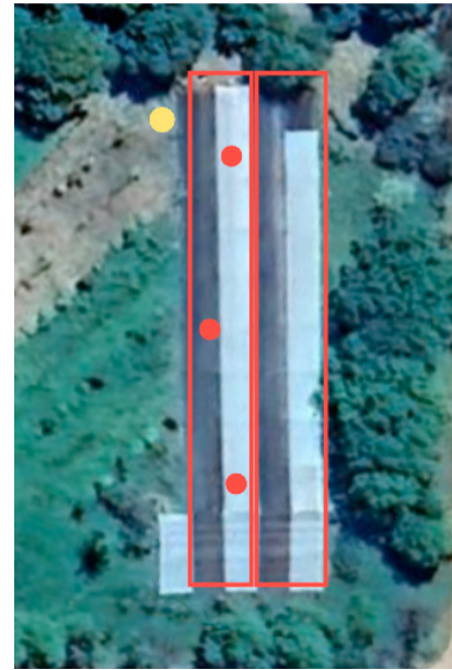
Fig. 2. Aerial view of the plot with semi-shade cover. The left side corresponds to the automatic subplot and the right one to the manual subplot. The red dots indicate the position of the 3 pure sensing nodes and the yellow dot is the control panel with sensing/actuation node.
