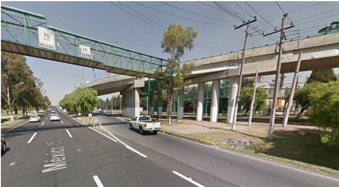
Fuente: Google Street View, Avenida Tollocan, Toluca 2014.
