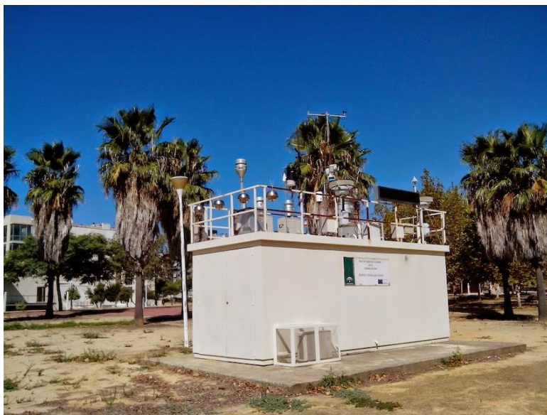
Fig.1.12.b. Monitoring station at the University of Huelva (El Carmen Campus).
