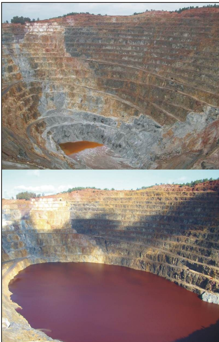
Figure 9. Atalaya open-pit before cessation of drainage pumpings in 2001 (up) and in 2014 (down).
