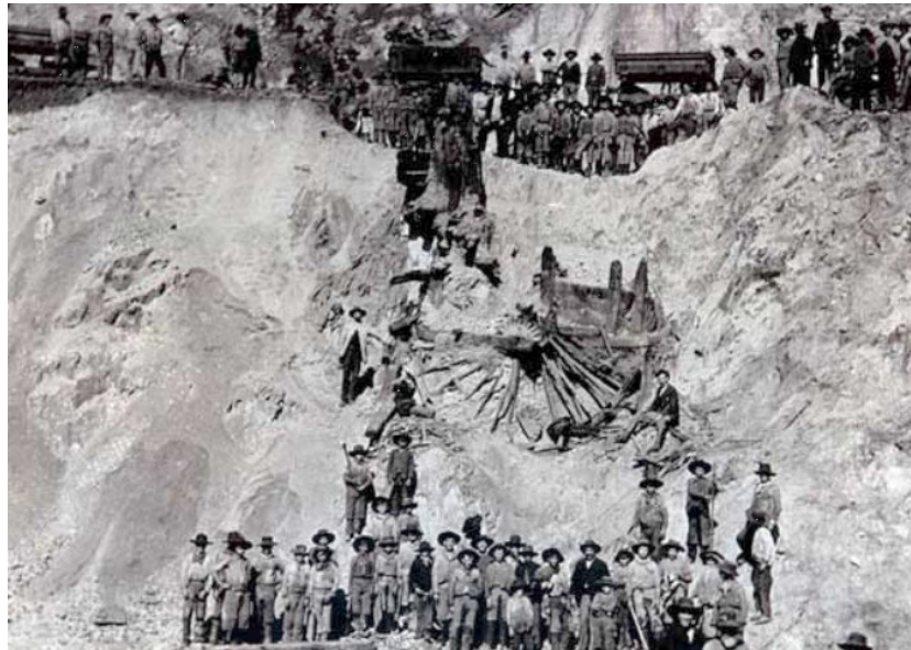
Figure 2. Roman wheel found in the early twentieth century in South Lode. It was part of a group of some 50 waterwheels, which could raise water more than 80 m to an adit (Río Tinto Mine Foundation).
