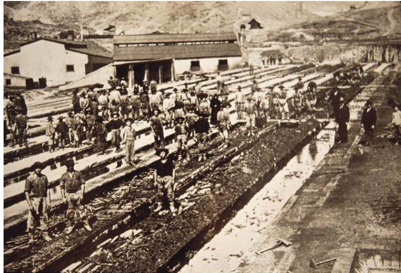
Figure 5. Channel systems for copper precipitation from acidic leachates in Zarandas-Naya zone at 1900 (Río Tinto Mine Foundation).
