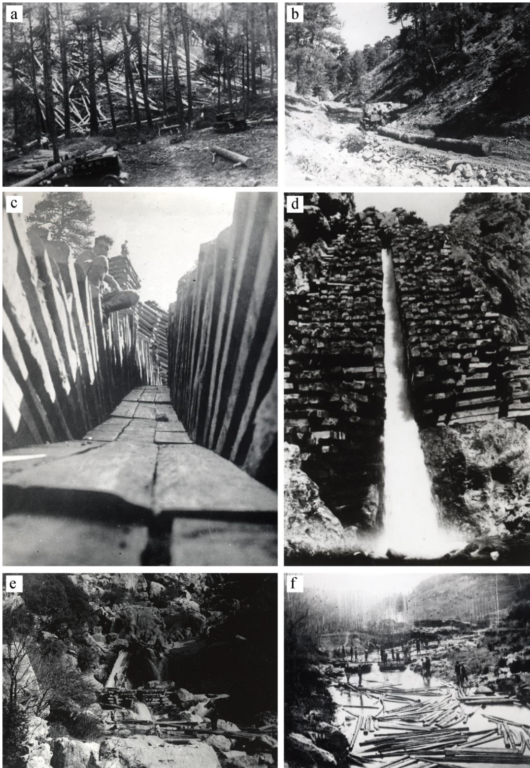
Figure 8. Sequence of production and transport of black pine ( Pinus nigra ) railroad ties from forests in the Cazorla Mountains (south of Spain) down to the Guadalquivir valley. This manner of timber transportation was used until the mid-20th century. Source photos: Archivo Histórico del Museo del Ferrocarril de Madrid - Fundación de los Ferrocarriles Españoles.
