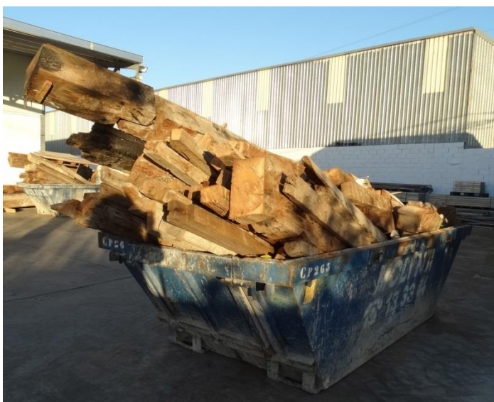
Figure 9. Roof timbers removed from an historic building in Andalusia, ready to be disposed. Photo: M. Domínguez Delmás.
